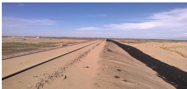
Fig. 1. Sandy drift of a railway track near the station Altynkol (Kazakhstan) (Photo: Mirakhmedov M., 2012)
