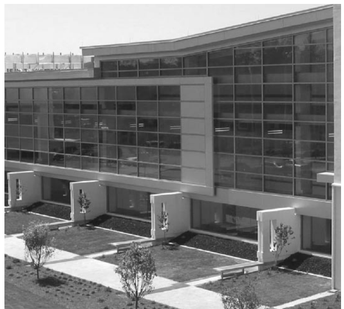
Fig. 2. New blood processing facility in Douglasville, Georgia.
