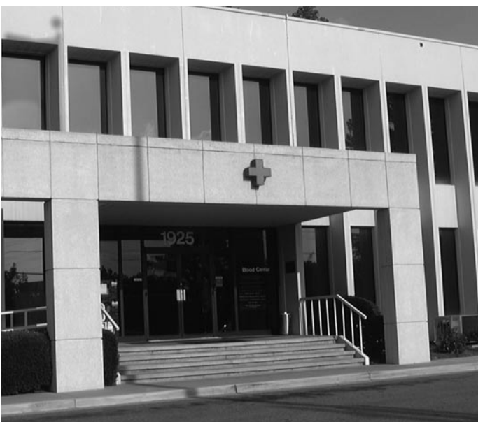
Fig. 1. Southern Region headquarters in Midtown Atlanta, Georgia (1965–2007).
