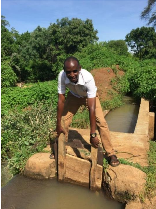
Figure 5-K: Steve demonstrates how the flow of canal water is regulated at the intake point.
