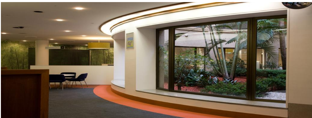
Figure 5.4 Parramatta Family Law Court Registry – New 'Sit-Down' Counters Without Safety Glass
