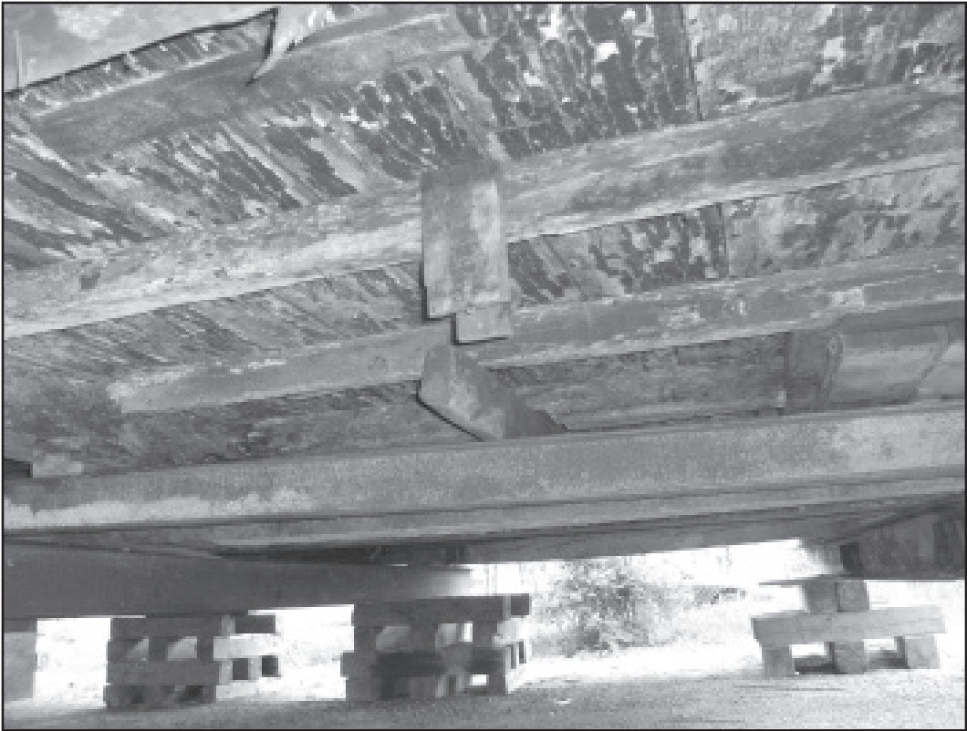
Figure 5. The sill and floor joists were excellent materials for sampling and dendrochronological analysis. (Photo by Jonathan Fowler, 2010.)
