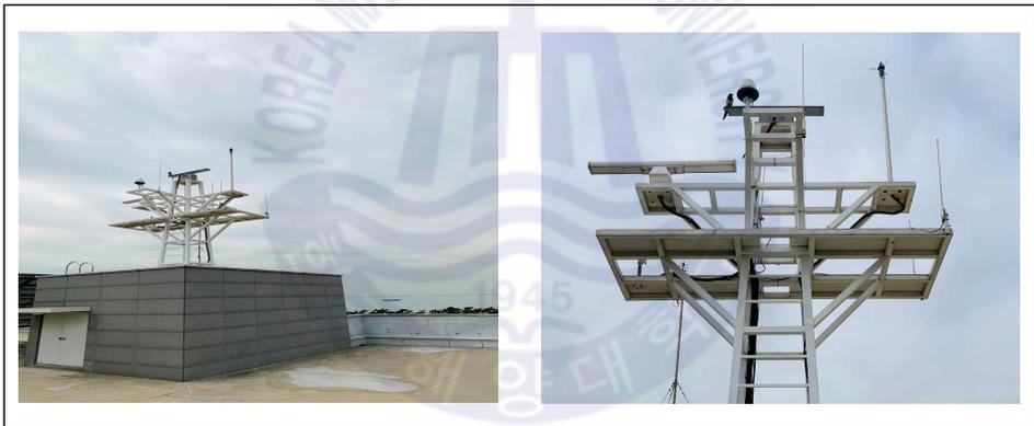
Fig. 3.1 Installed AIS receiver
