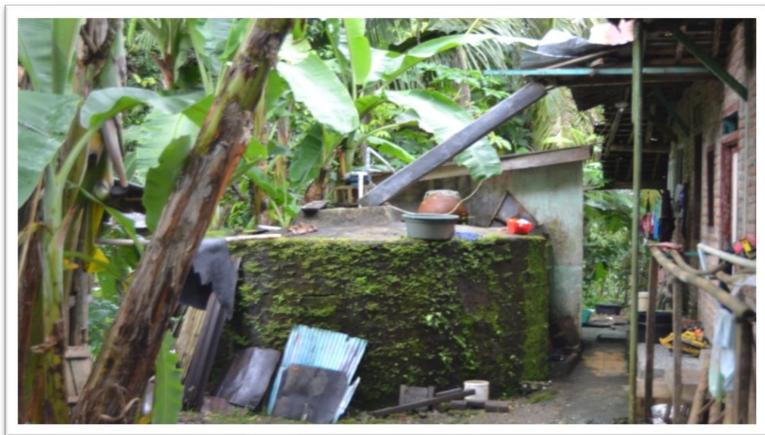
Picture 2.8: Big barrel used to collect water during the rainy season (Photo taken on 29/01/2017)
