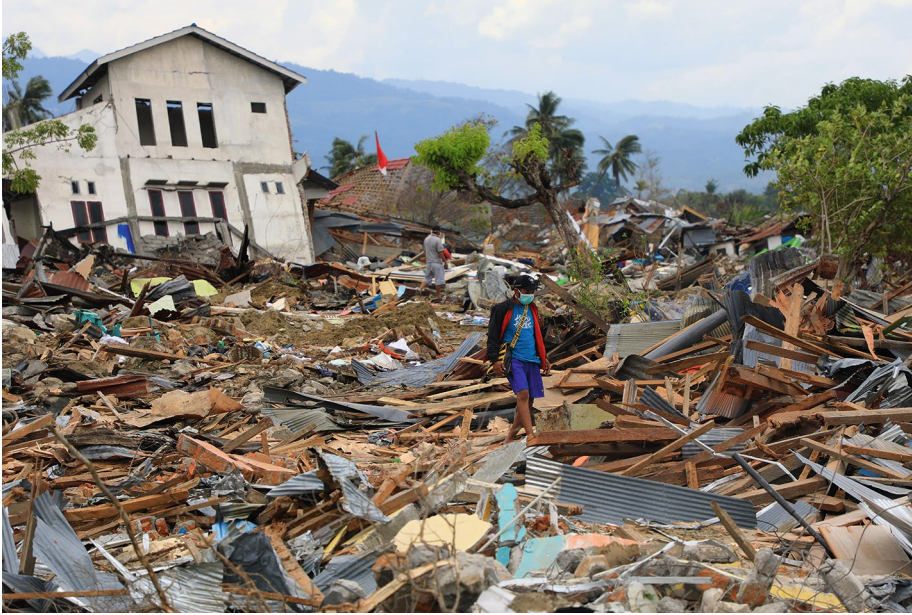
Fig. 1 | Destruction by liquefaction, Petobo, Palu. Bradley and colleagues 4 and Watkinson and Hall 5 conclude that the landslides on very gentle slopes were made possible by wet rice cultivation that led to water-saturated soils and liquefaction upon shaking by the M_w 7.5 earthquake. Other regions in Asia could be prone to similar hazards. Credit: Pacific Press Agency / Alamy Stock Photo
