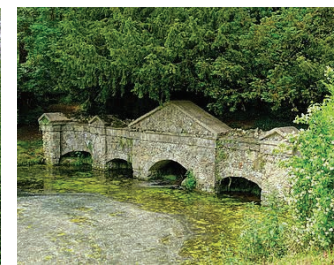
The Shell Bridge William Kent, 1739
