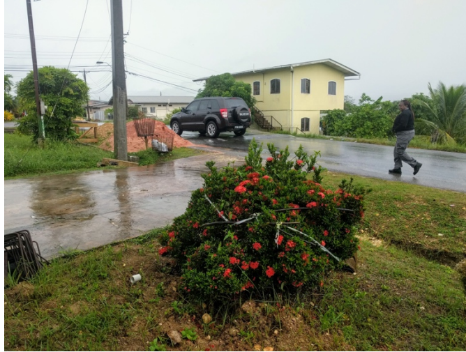
Image 12: Construction material for the drain outside Peter's house
