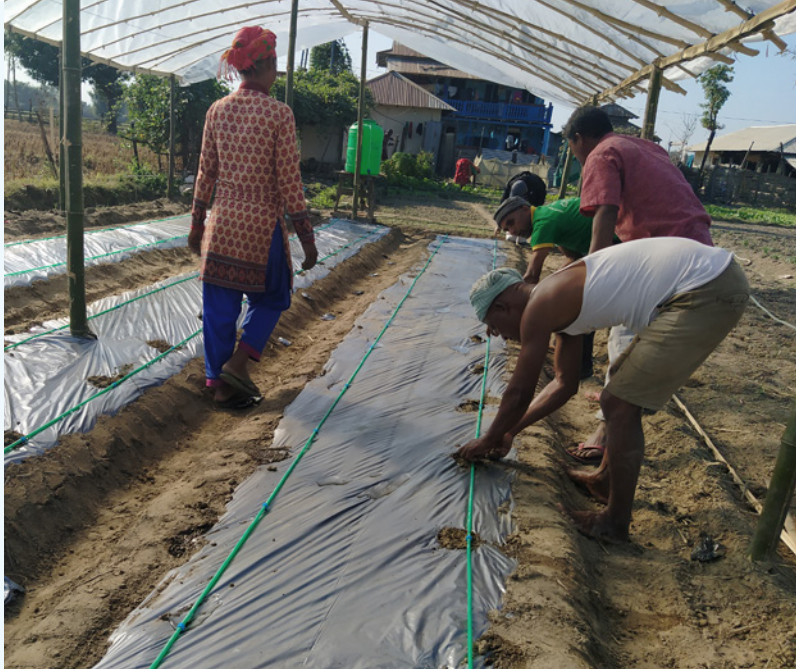
Farmer installing drip irrigation system along with mulching in the field. Photo: Sagar GC, LI-BIRD
