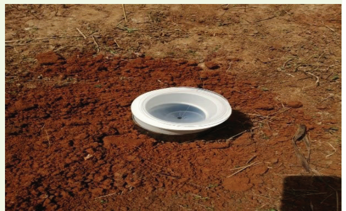
Fig 4.0. Picture of an installed rain gauge at Abotareye in the Cope Zone for PBC
