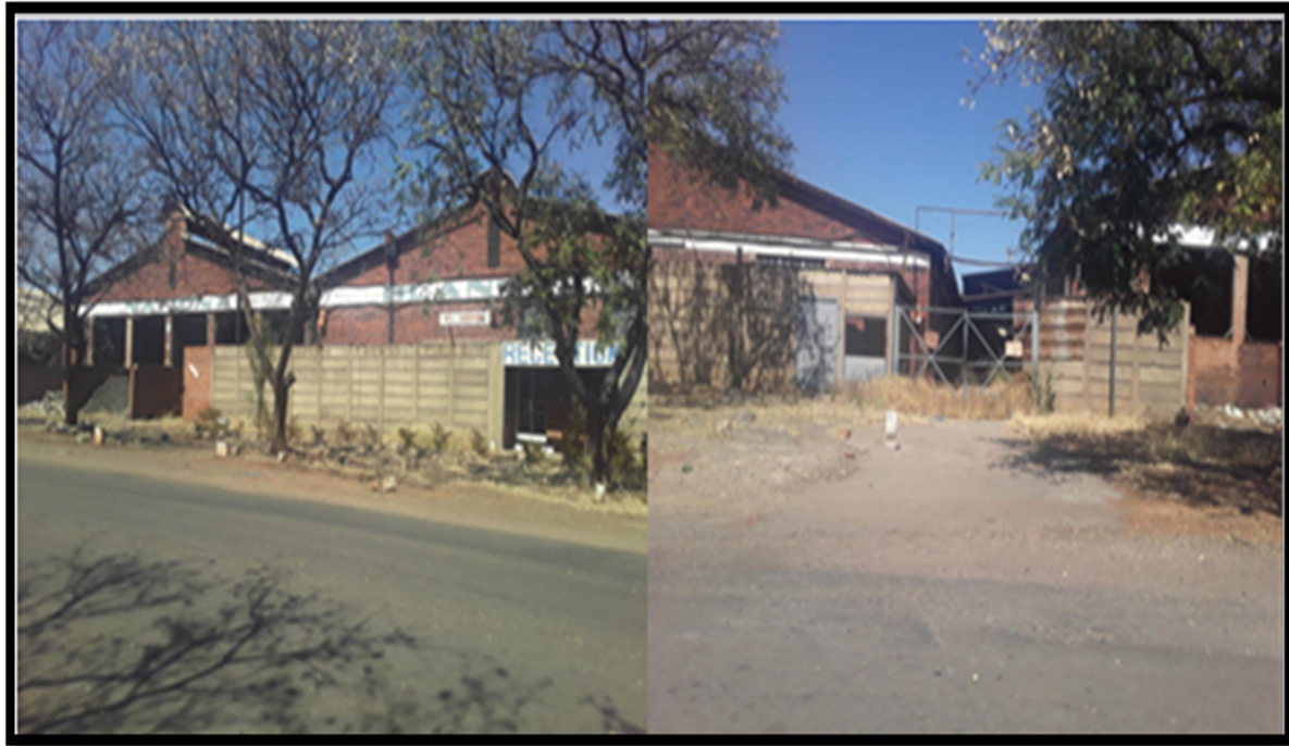
Figure 6.3 Vacant industrial building in Bulawayo
