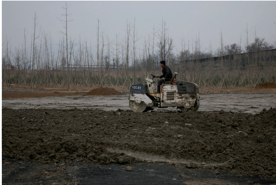
Figure 6. Use a tractor for site preparation.
