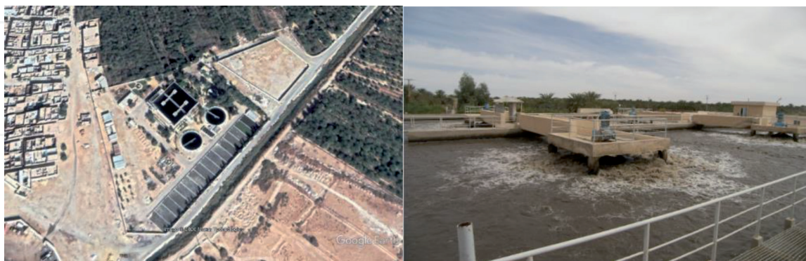
Figure 14. Touggourt wastewater treatment plant.
