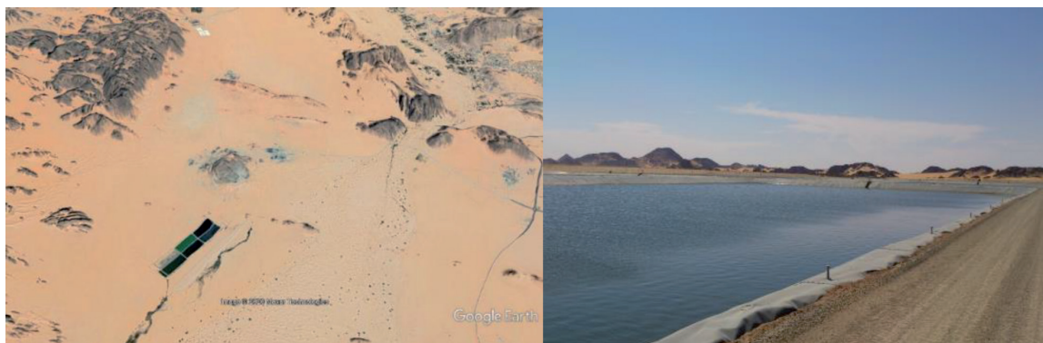
Figure 4. Djanet wastewater treatment plant.
