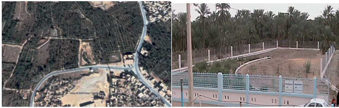
Figure 12. Temacine wastewater treatment plant.
