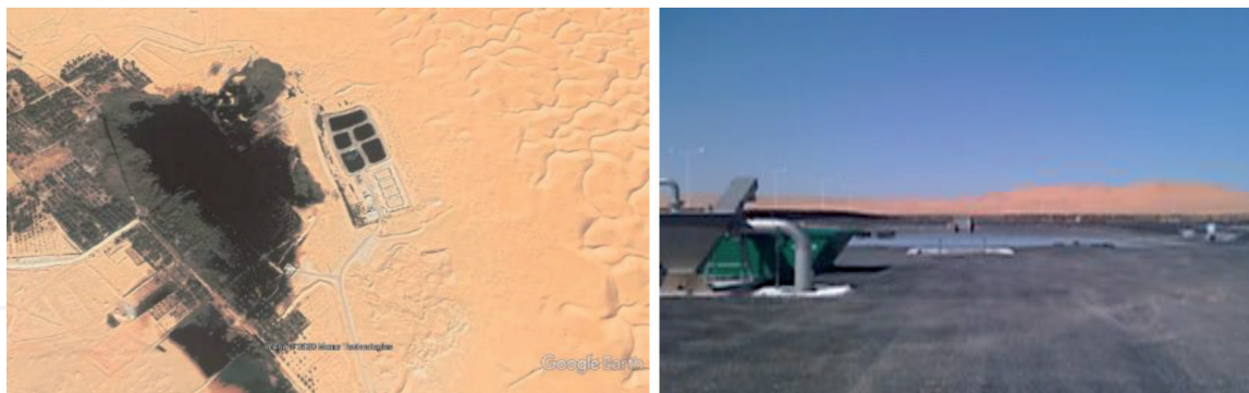
Figure 8. Sidi khouild wastewater treatment plant.
