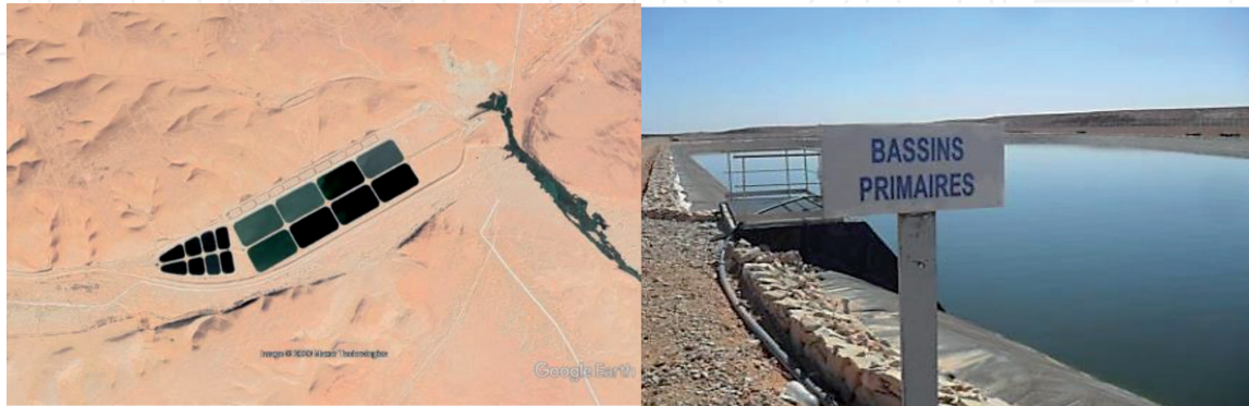
Figure 2. Ghardaia wastewater treatment plant.
