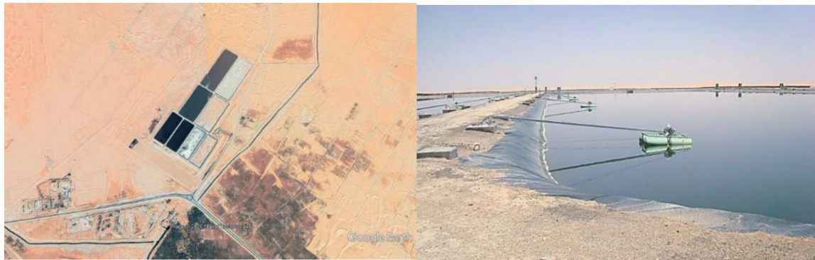
Figure 6. Ouargla wastewater treatment plant.
