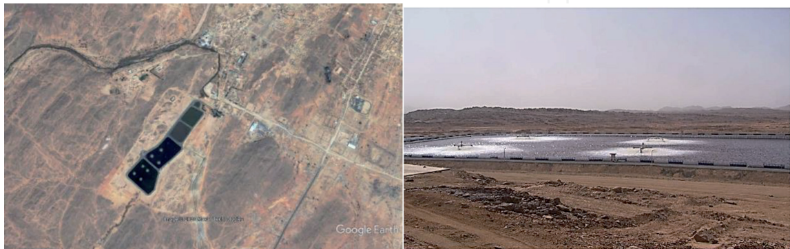
Figure 7. Tamanrasset wastewater treatment plant.
