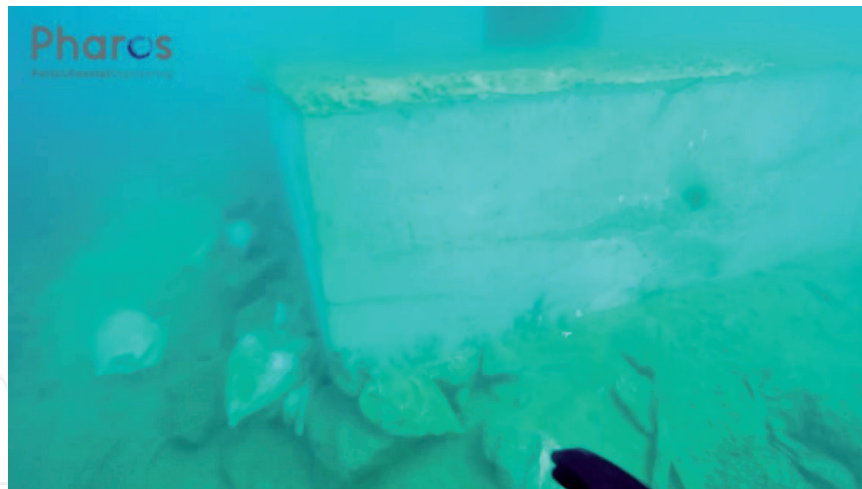
Figure 25. Corner detail of the Duke of Alba's foundation slab (Port of Naos).
