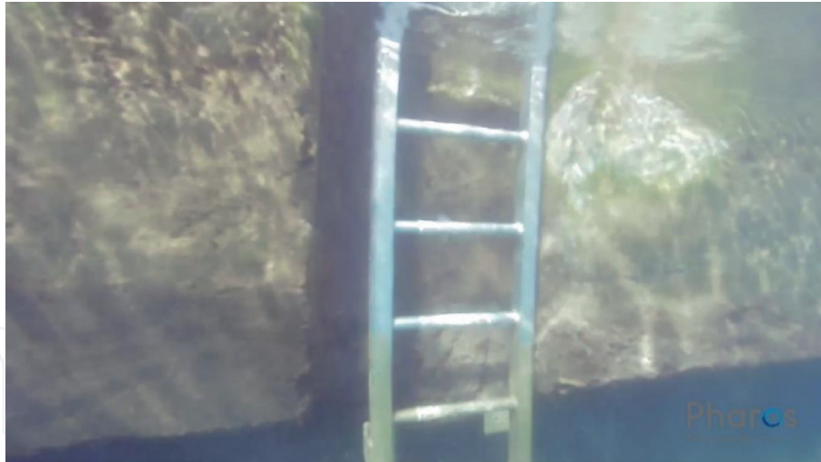
Figure 8. Lip finish of superstructure in submerged area.
