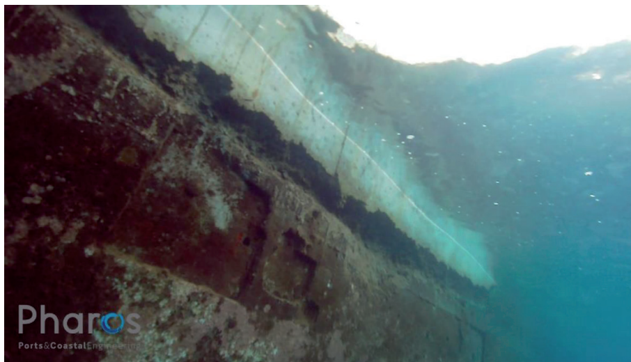
Figure 14. Ramp repair area.
