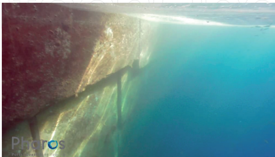
Figure 15. Vertical face of the ramp.
