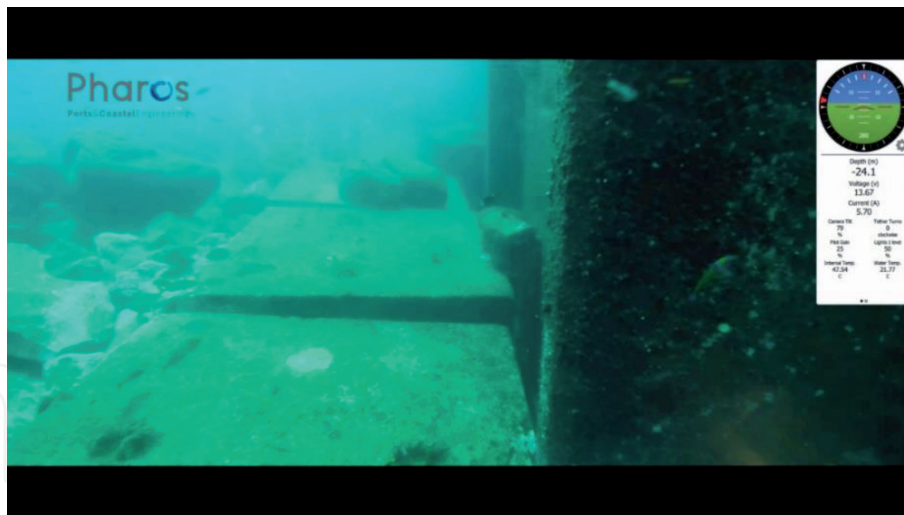
Figure 18. Guard concrete blocks on the foundation bank of the external dike.
