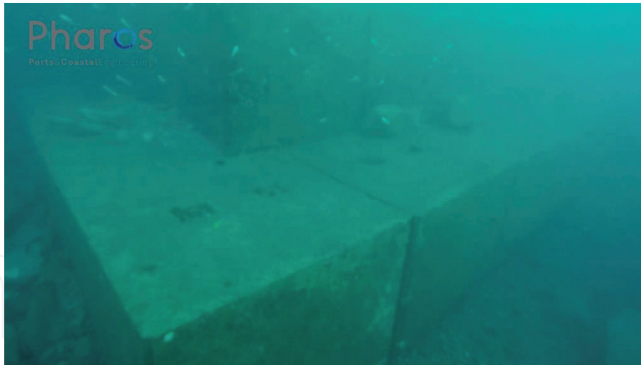
Figure 13. Detail of the foundation of the ramp.
