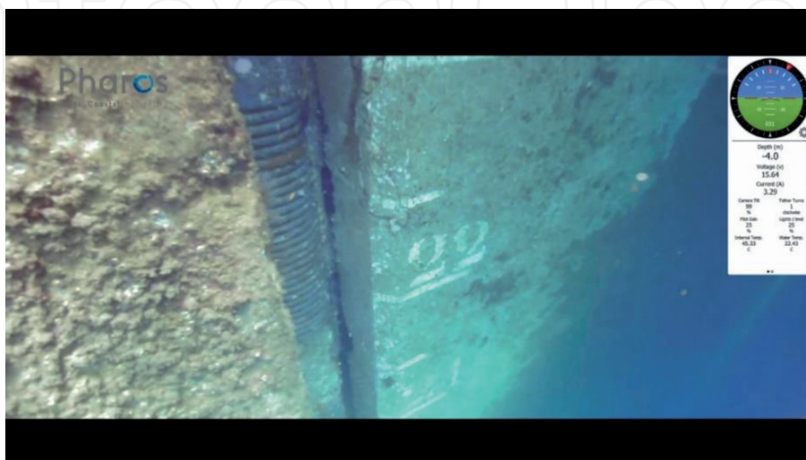
Figure 17. Detail of depth markers on the facing of concrete quay blocks and joint.
