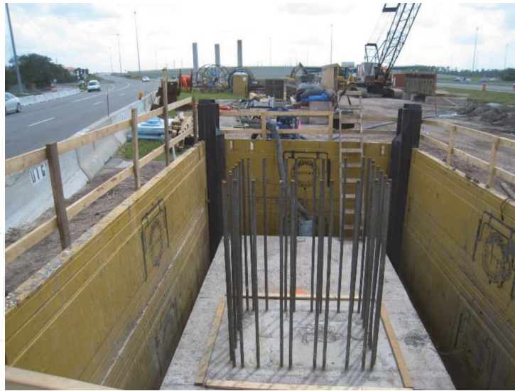
Figure 3. Bridge footing for monitoring in Orlando, Florida.
