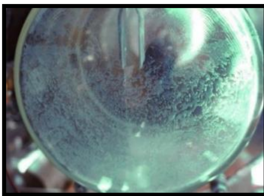
Figure 4-12 Formation of scale on the reboiler wall
