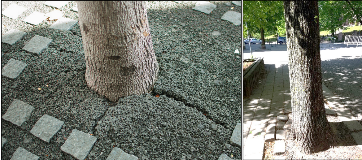
Figure 19 Examples of compaction over the root extent. The roots are limited in four directions: there are 100 % and > 90 % of compaction over the root extent, respectively. Picture 1 (“ Tree v concrete ”) by Ruben Schade on www.flickr.com (CC BY-SA)
