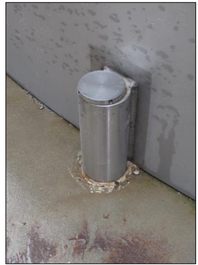
(c) Energy dissipation devices used for anchoring 240 kL tank
