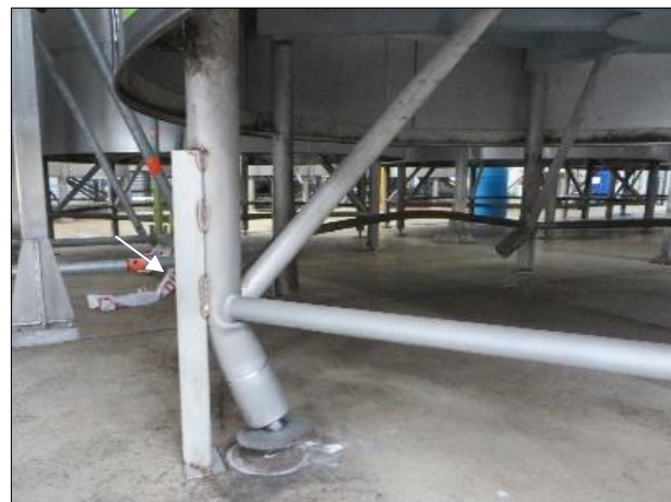
Figure 21: Example of welded steel angle temporarily used to support legged tank.
