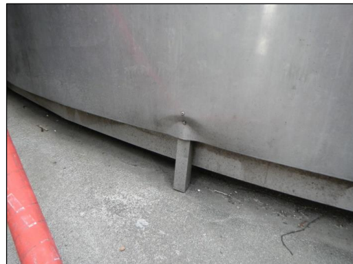
(b) Tank 400 kL- minor damage to the skirt
