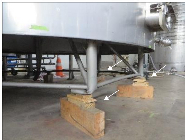
Figure 20: Example of wooden blocks temporarily used to support legged tank.
