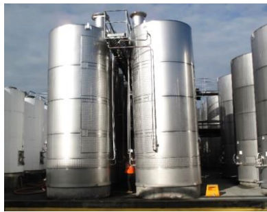
(b) 150 kL tanks, after 2016 earthquake
