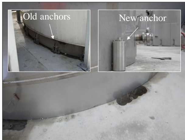
(a) Anchor bolt replacement for tank with 225 kL capacity
