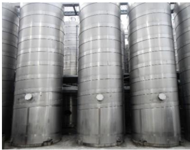
(a) Tanks of unknown tank capacity, after 2013 earthquakes
