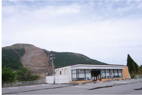
Fig. 11.2 A photograph of Kurokawa's landscape after the Kumamoto Earthquake: large cracks in the ground are evident
