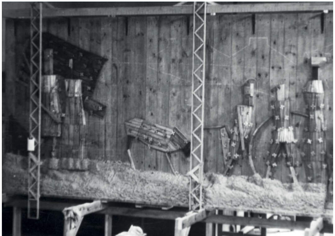
Figure 11.9: C1. Hendrik Ploeger. Wooden armature for full-scale clay relief of Descent , 1943–45 (courtesy of Kirchhoff files; photo Alan Yates)
