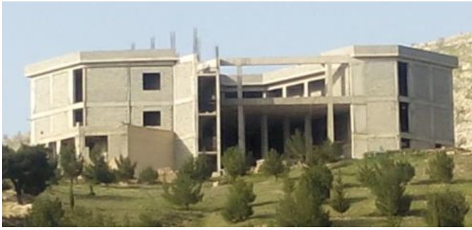
Fig. 1. Concrete structure erected with diaphragm Cellular Concrete Block (Photo by Authors)
