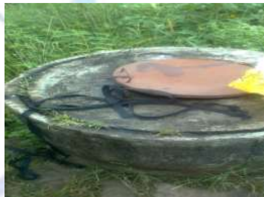
Well D: An unraised well with metal cover surrounded by grasses
