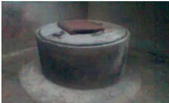
Well A: A raised well with metal cover and with openings at the sides
