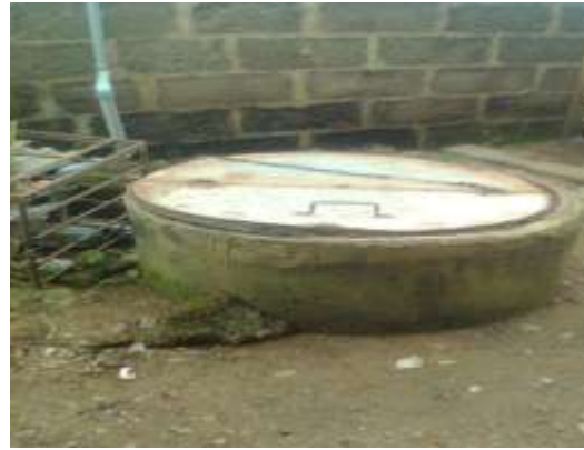
Well H: An unraised well with metal cover with an untidy environment
