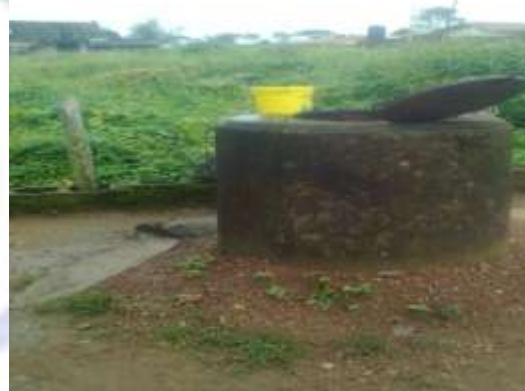
Well J: A raised well with metal cover
