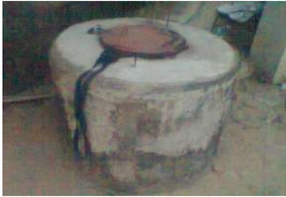
Well G: A raised well with metal cover
