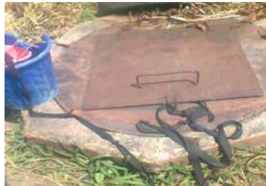
Well B: An unraised well with metal cover surrounded by grasses
