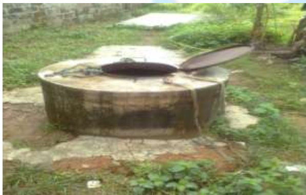
Well C: A raised well with metal cover
