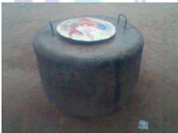
Well E: A raised well with metal cover
