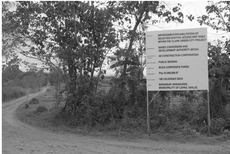
Fig. 7. CGC Roadworks in Brgy. Aranguren, Capas, where a farmers' barricade was staged in April 2015
