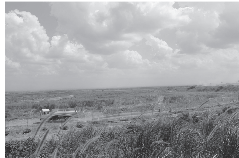
Fig.2. Ongoing Construction of Alviera as of February 2016
