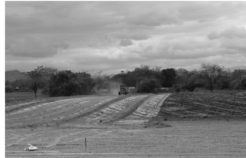
Fig. 4. Construction of Clark Green City as of February 2016 Source: Author
