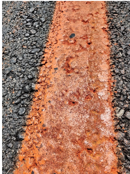
Figure 4.6 Close-up of High-Build Paint
