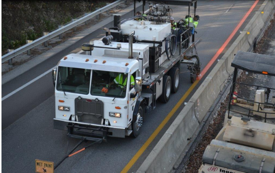
Figure 4.1 Initial Installation of Orange Paint
