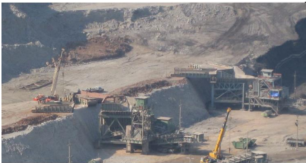
Figure 2-4- A SMIPCC system in an open-pit mine [48]
