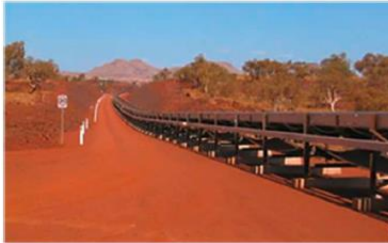
Figure 2-9. Semi fixed conveyor belt [7]
