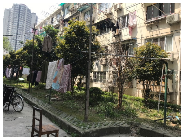
Figure 2. Real photos of Workers' New Village, Shanghai
