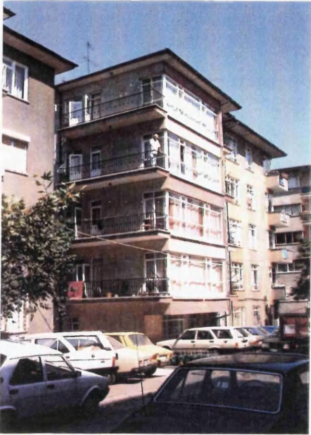
Photo 1- Buildings on plots 2685/10, 12 and 11 (left to right)
