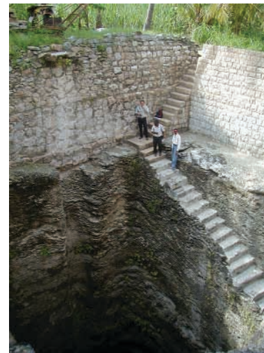
Community management of groundwater resources in rural India: large dug well in Tamil Nadu, India, which has had to be deepened due to a regional decline in groundwater levels.
