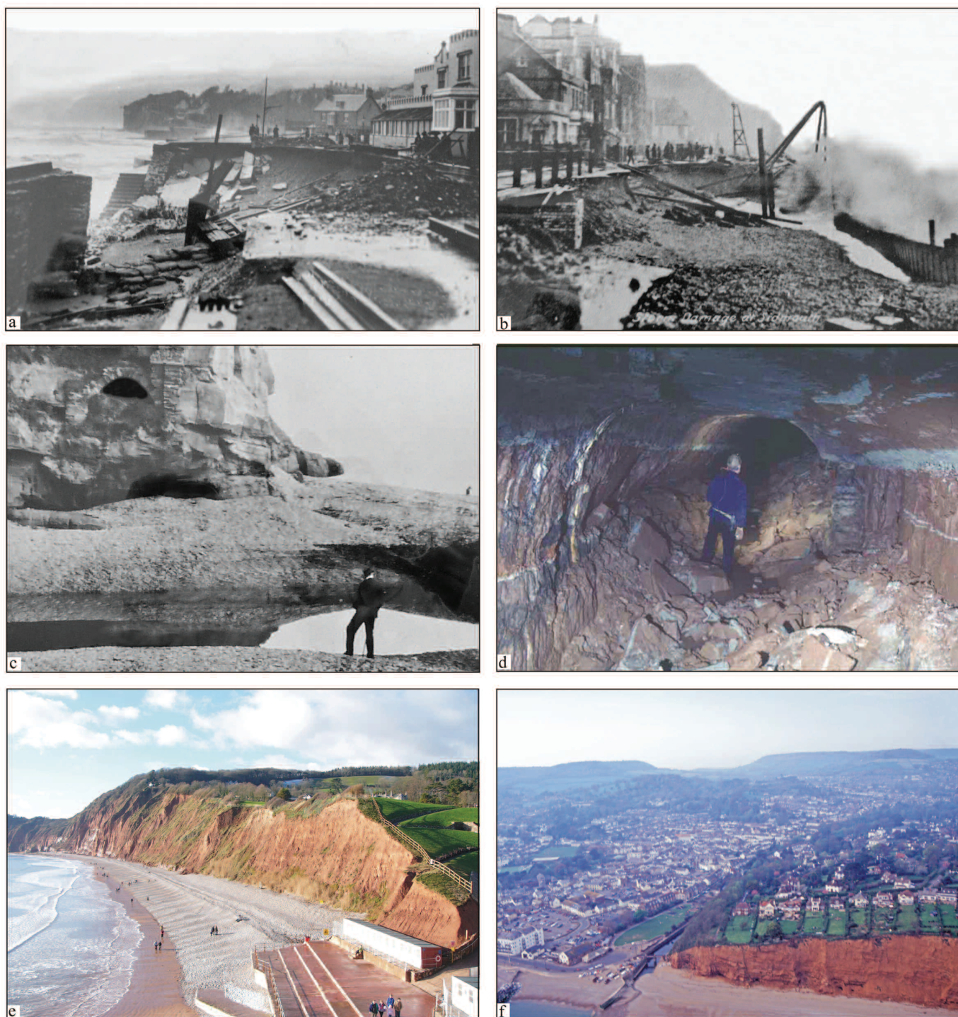
Figure 3. (a) Storm damage to the sea wall and the Esplanade in January 1925, view west. The western pier (The Hump) and Connaught Gardens Cliff are visible in the background. (b) Storm damage in January 1925, view east. The storms persisted for several days. Emergency repairs including the installation of sheet piling (bottom right) were carried out at times of low tide. (c) The western end of the railway tunnel in 1910. The River Sid percolated out through the beach gravels, as it did in October 2011. (d) View east inside the tunnel in February 2004 about halfway along its original length. The tunnel is in the lowest part of the Sidmouth Mudstone Formation at this point. Parts of the rounded arch shape of the tunnel are still well preserved. Almost all the roof falls are joint-bounded rock-block failures in thickly and thinly bedded mudstones. Photograph by and courtesy of Peter Glanwill. (e) View west towards Peak Hill from the top of Jacob's Ladder, December 2004. Beach gravels, almost all chert and flint derived from the Upper Greensand and Clay-with-flints, are banked up against the 1934 esplanade. (f) Oblique aerial view of the outfall of the River Sid, May 2005. Low tide at a time when the level of the beach gravels east of the river was high. Photographs a, b and c courtesy Sidmouth Museum.
