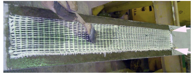
Figure 5: Application of textile sensor on the surface of reinforced concrete element.
