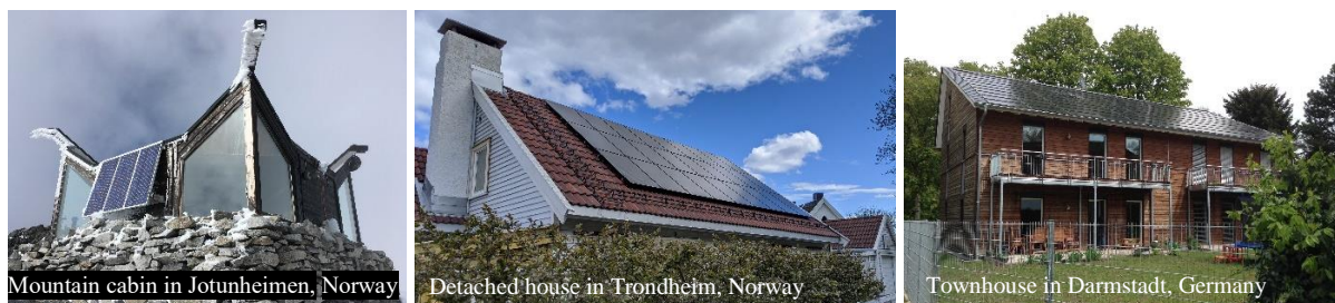
Figure 1. Off-grid PV system installed on the façade of a mountain cabin, building applied PV (BAPV) system attached on the roof tiles, PV tiles system (BIPV) integrated into the roof. (Source: authors’ photos)
