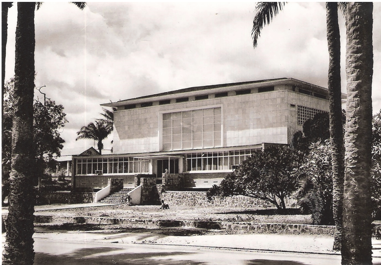
Figure 13. BCB Headquarters in Stanleyville. Source: www.delcampe.be
