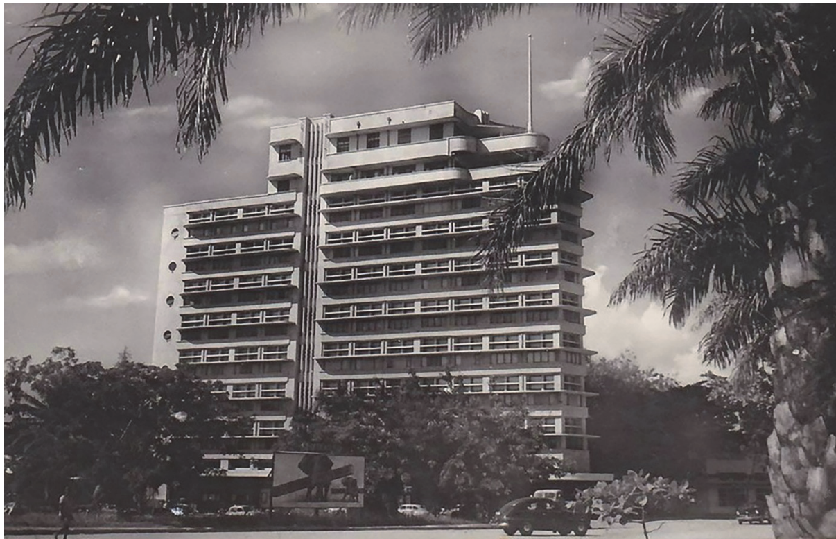
Figure 1. Forescom Building in Kinshasa, 1946. Source: www.delcampe.be
