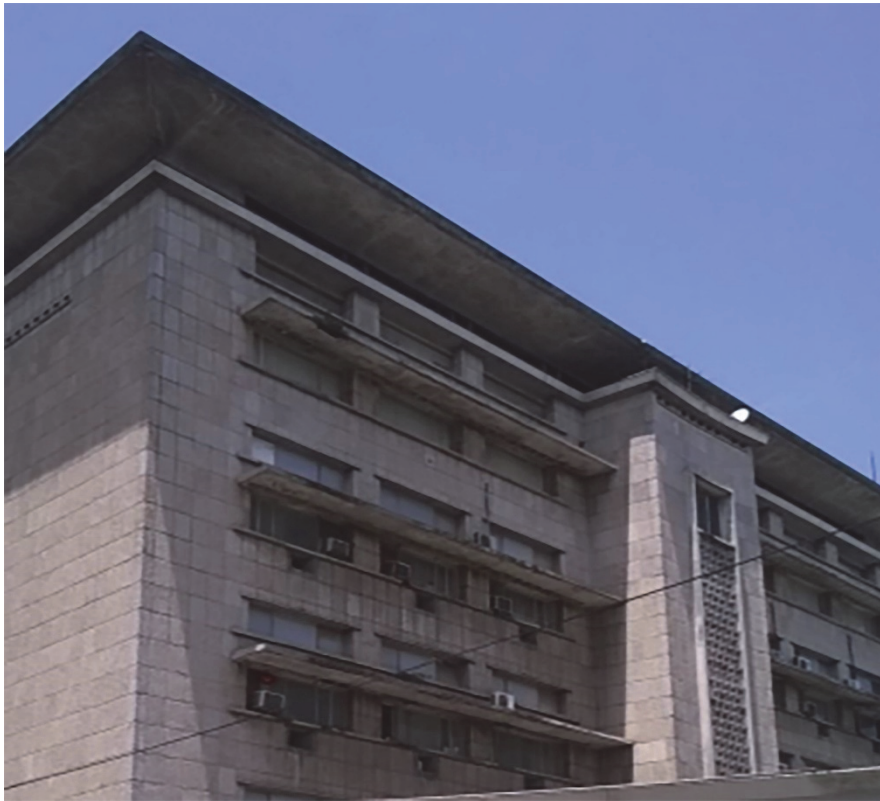
Figure 6. BCB building south elevation with overhanging slabs and lift ventilated trough claustras. Source: picture by Alexis Tshiuza (2016)
