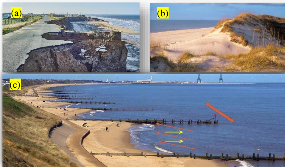
Figure 1-1: Coastal erosion (a) Offshore (b) Onshore (c) Alongshore
