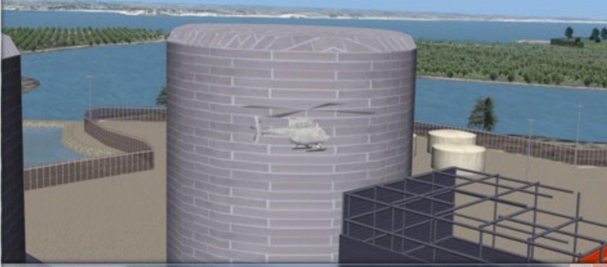
Figure 23 – SFP Replenishment by water bucket drops (Davis, Proctor et al. 2016)
