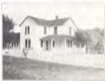
NO. 2 - B. STANLEY'S WHITE BRICK HOUSE, FRONT AS TO BRIDGE AND SIDE
