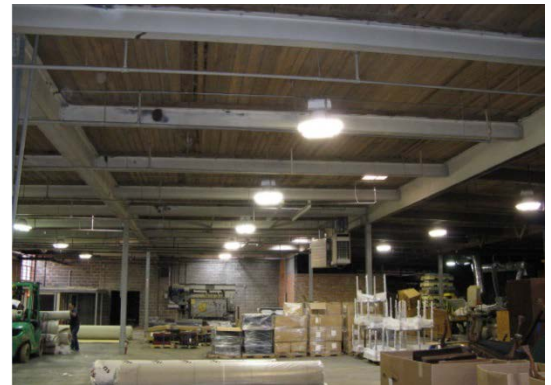
Upper Level – Right Side of Building
