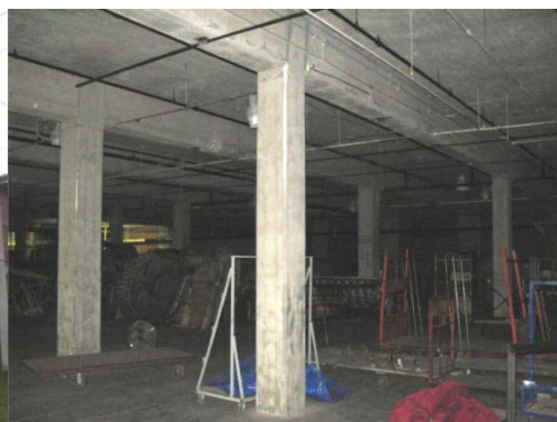
Lower Level – Concrete Columns
