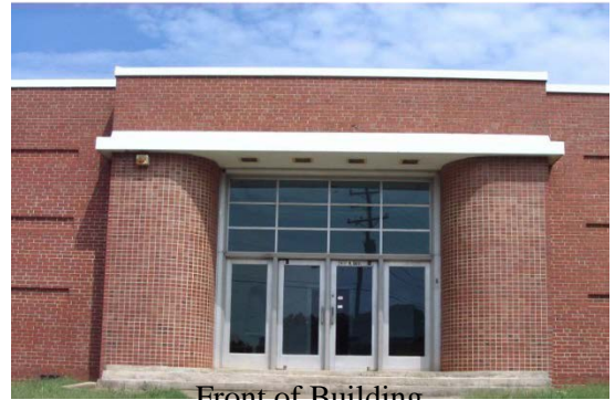
Front of Building
