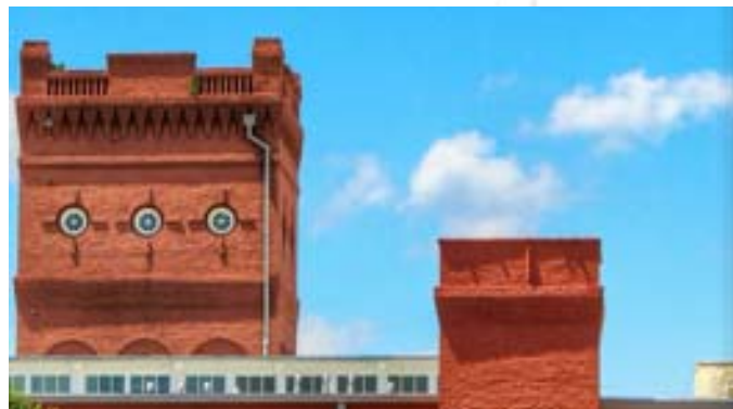
Highland Mills Lofts
