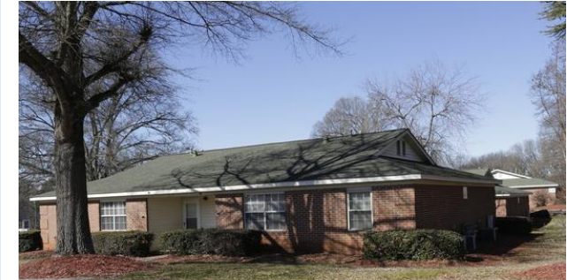
801 W Washington St – 1.1-mile from site
