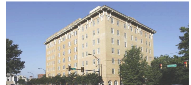
201 W Washington St – 0.7-mile from site
