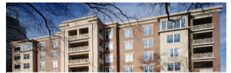
0.3-mile from site
