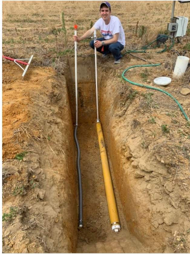
Figure 2.5. Devices 3.2 and 3.3 Being Installed in the Field
