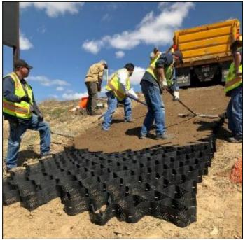
**Figure H2**. DEN Field Maintenance personnel moving the topsoil down the slope to fill GEOWEB cells.
