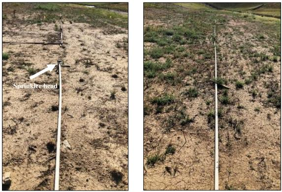
**Figure 25**. Simple irrigation system used to ensure grass establishment at DEN demonstration sites. Left picture – hose connection located at the middle point of the 250 ft PVC pipe. Right picture – PVC pipe runs down the middle of the site.
