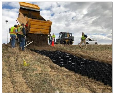
**Figure H1**. Black material is the GEOWEB system laid and stretched out along the side of the slope. Topsoil was dumped at the top of the slope to fill GEOWEB cells.
