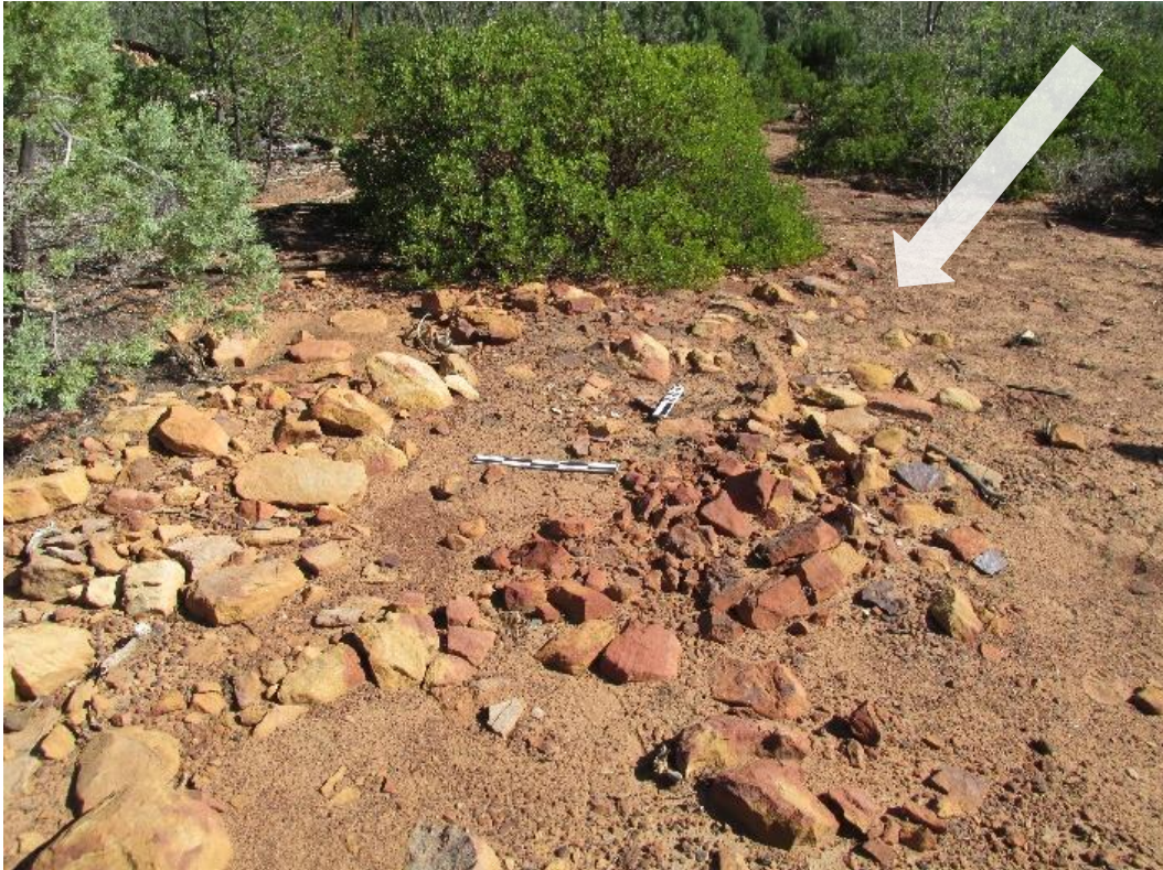
Figure 6.12. Dislocated and dispersed masonry elements from roomblock feature at site 07-0612. Pre-fire records indicated that these features were intact and standing.
