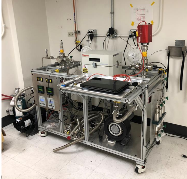
Figure 3-47 TDS equipment located in LAMDA at ORNL.
