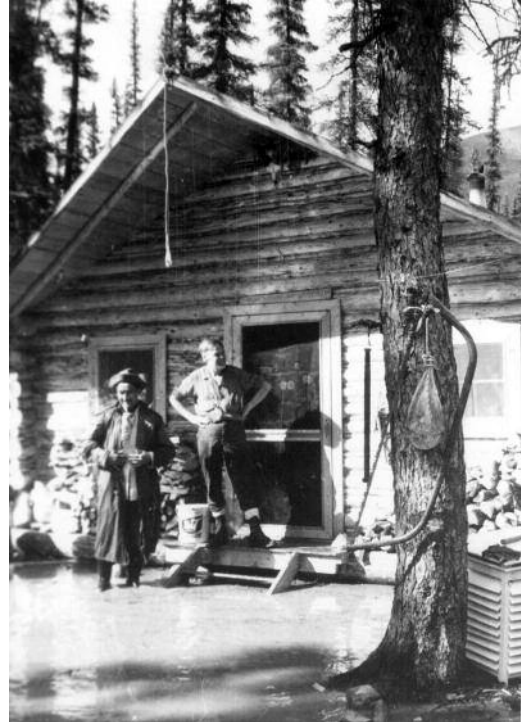
FIGURE 7. Bill Cody (right) and Dene Gabe (left, standing in floodwater) at the log cabin as floodwaters rose to the front door. The water eventually rose to at least the level of Bill's waist. Keele River, Northwest Territories, 1970. Photographer unknown.
