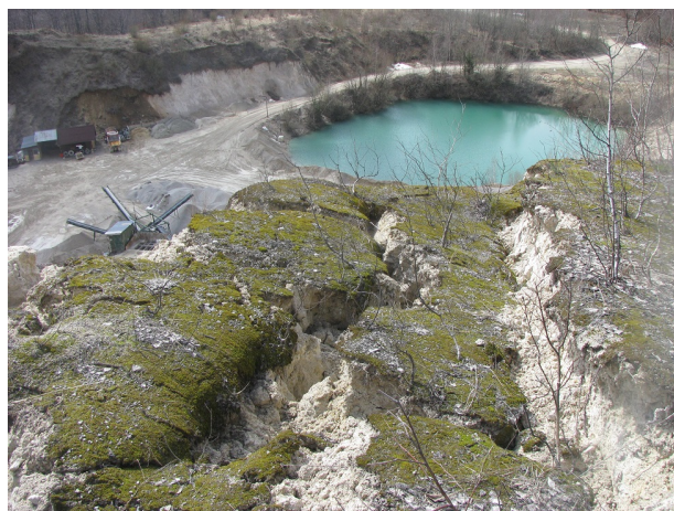
FIGURE 7. Cracks above the front of the rockslide in the central part near the point 640
