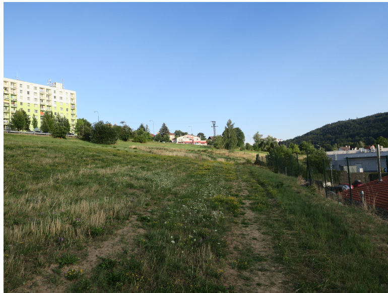
FIGURE 1. The slope above the gabion support wall, a car park with a shop (right)
