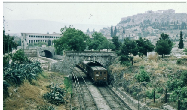
FIGURE 3. Original Athens metro line after doubling of the track [4]
