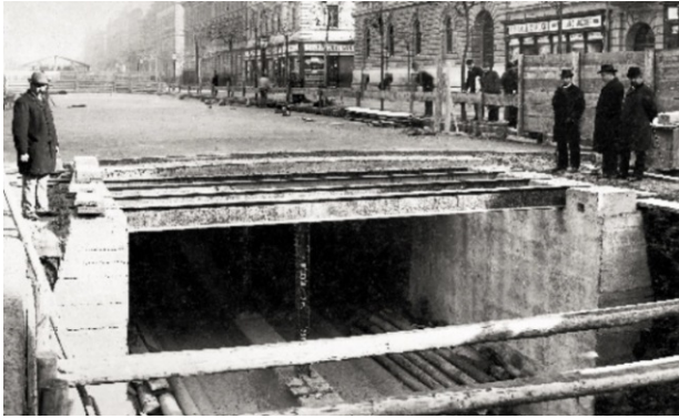
FIGURE 5. Földalatti under Andrassy Avenue [6]
