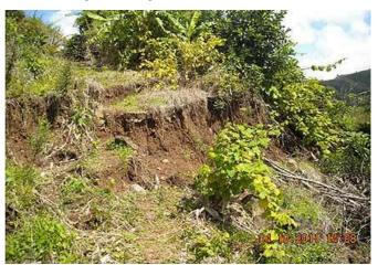
Figure2: Slope failures along cut mountain slopes of Terre Rouge Verdun Link Road
