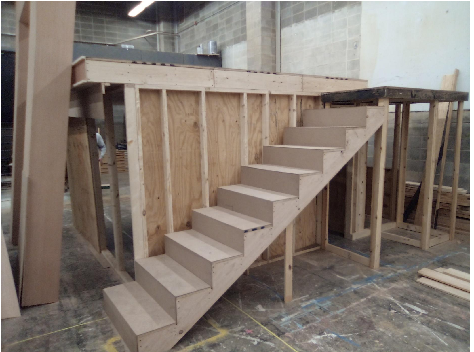
Loft with escape stairs
