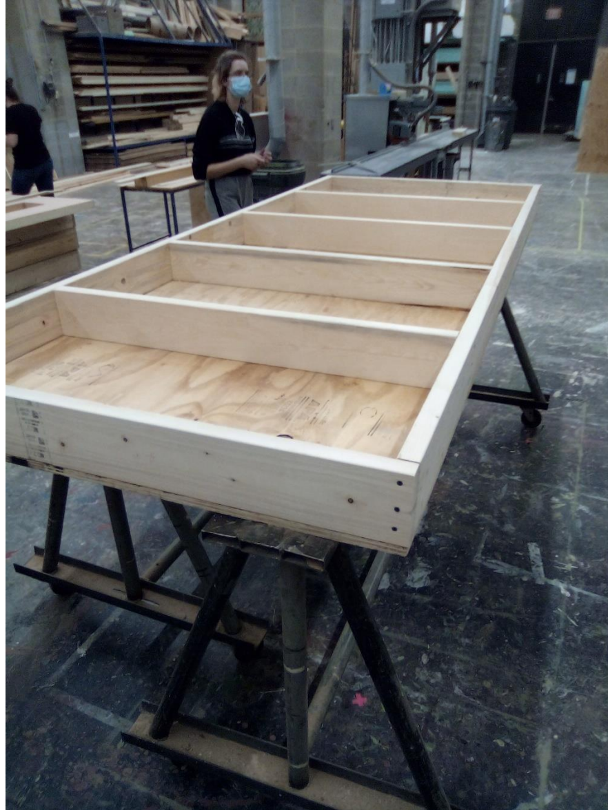
Ten-foot platform for catwalk construction
