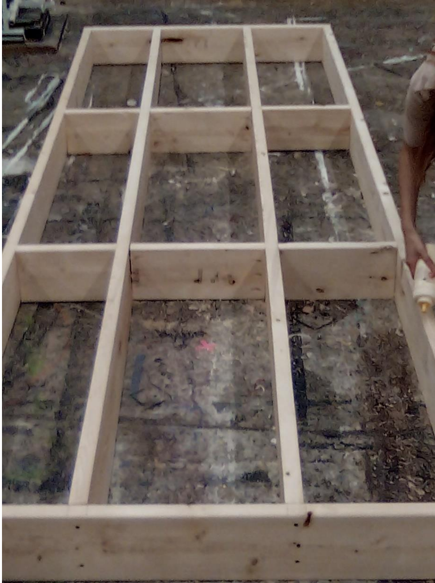
Loft deck platform frame
