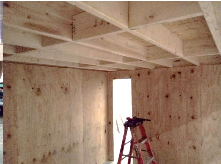
Figure 5.3: Deck Under side
