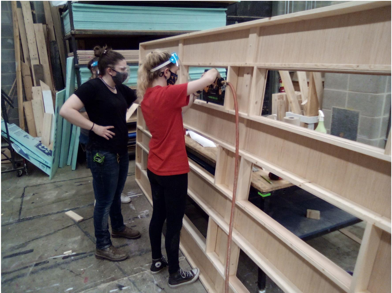
Students building abandoned building
