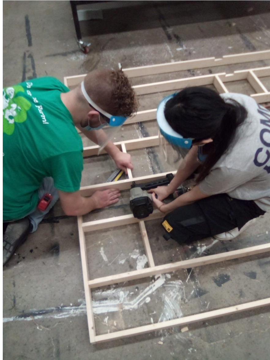
Stagecraft students building abandoned building
