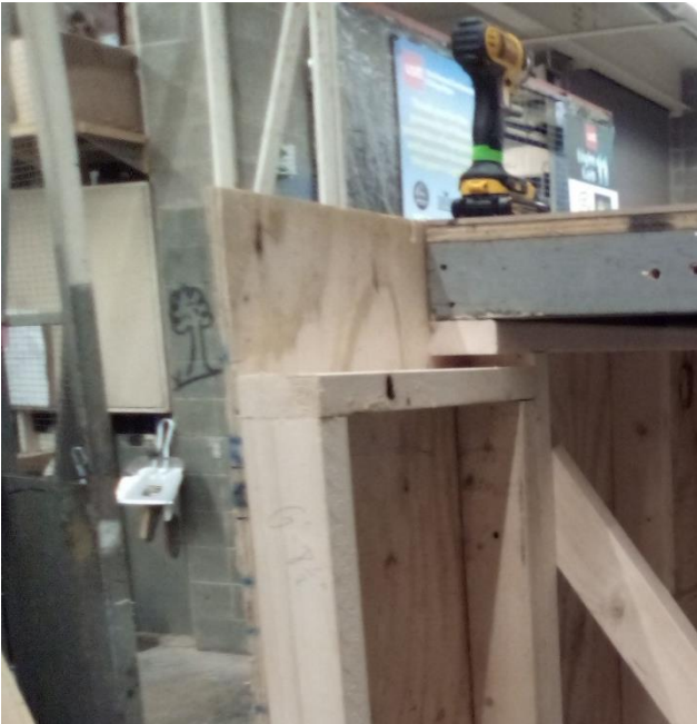
Figure 4.2: Stud wall Repair
